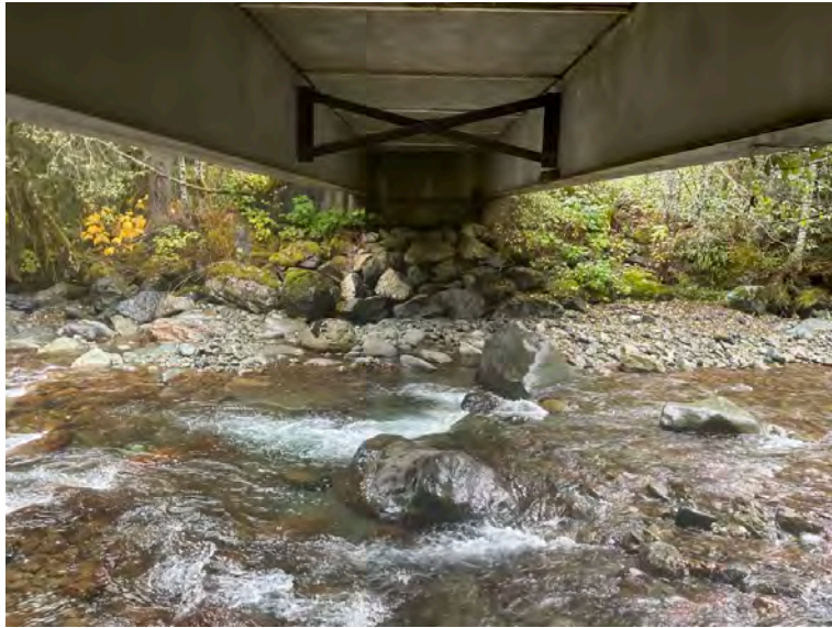
Right Bank Abutment when facing downstream
