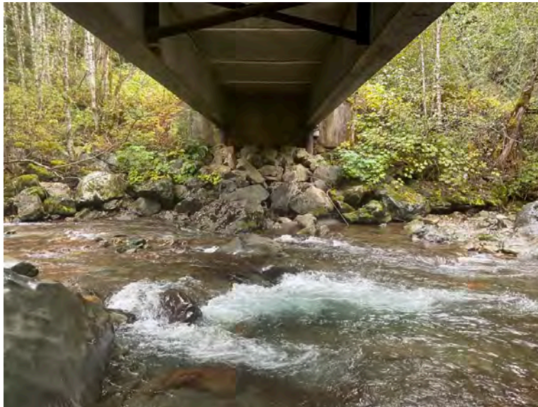
Left Bank Abutment when facing downstream
